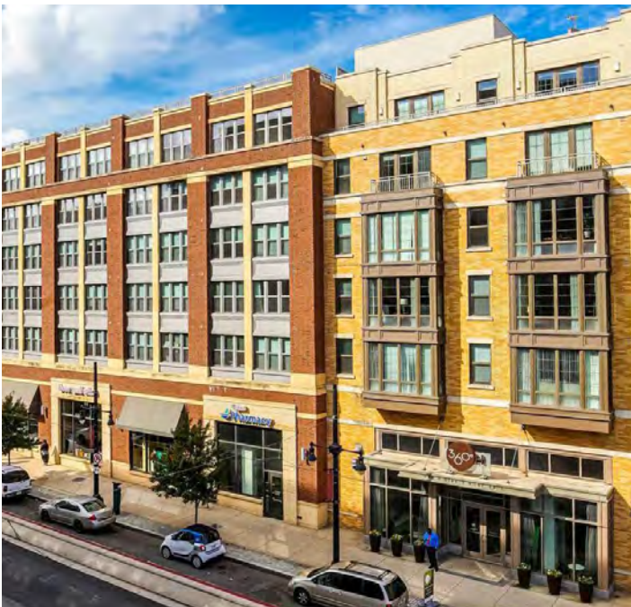
Figure 5.1.11 (a) Appearance of Two Buildings
