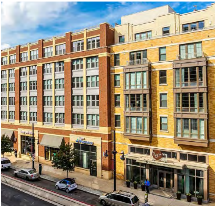
Figure 6.2.9 Appearance of Two Buildings
