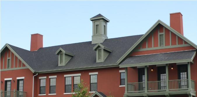
Roof Materials: Asphalt Composite Shingles
